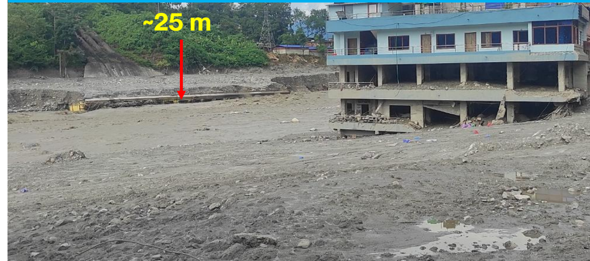
B) Raised river channel with reference to Hydro Station at Dhunge Bazaar
